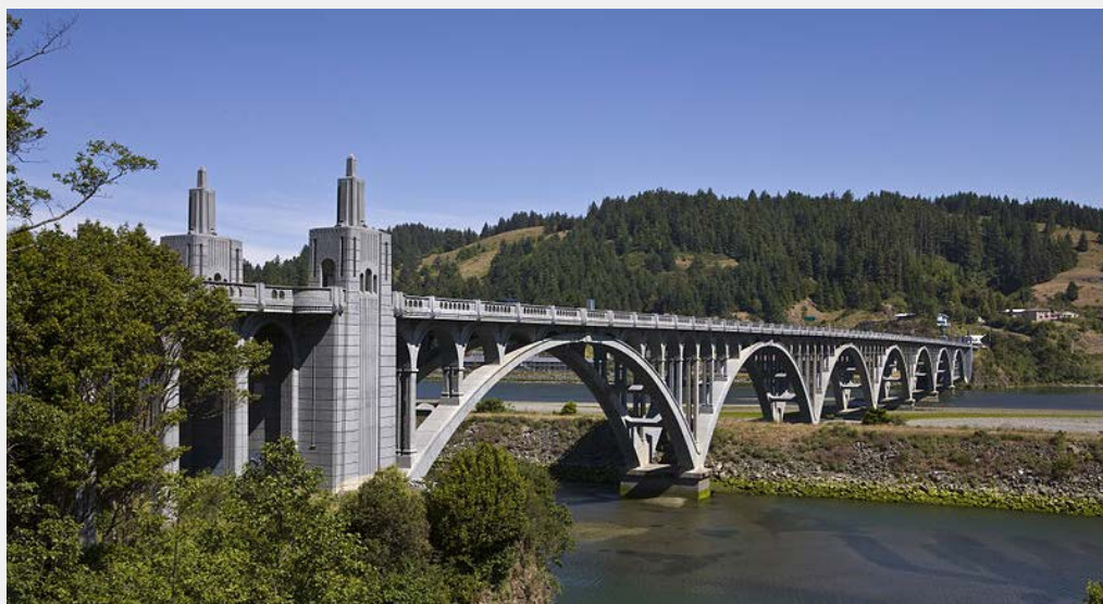
The Isaac Lee Patterson Bridge. Image source: Wikimedia Commons.
